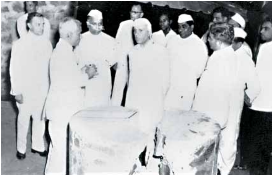
With Prime Minister Pandit Nehru laying foundation stone of Koyana dam in 1962
