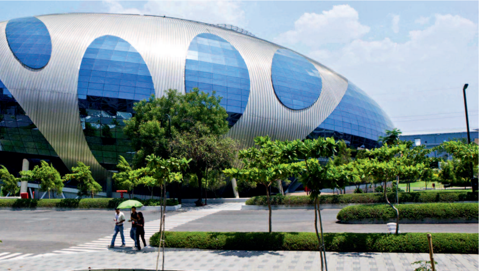
(Clockwise from above) Infosys office at Hinjewadi, Magarpatta and EON IT Park at Kharadi, in Pune
