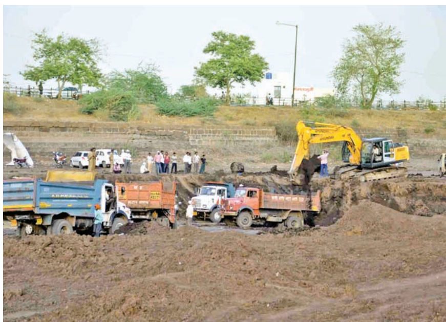
Desedimentation work at Bindusara lake
